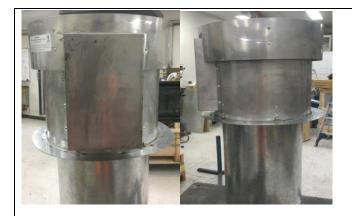
Rooftop fan module – Terminal must be installed with clearances as specified by AS/NZS 5601.1 Clause 6.9.3
