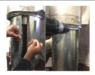
Flex collar and fit around the access panel. Socket the collar all the way up close to the air intake slots Ensure there is a rubber seal top and bottom of the collar.
