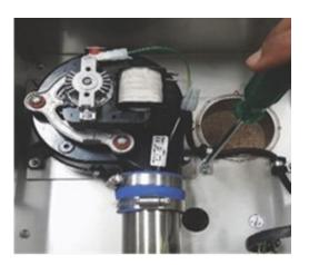
Push fan terminal into position. And affix to wall. Uneven or rough surfaces may require sealant along top and side gaps.
