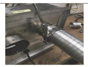
Slide flue onto connection spigot fully. Tighten clamp fully. Wipe excess silicon, visually check connection to ensure connection is fully sealed.
