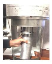
Slide flue onto connection spigot fully. Tighten clamp fully. Wipe excess silicon, visually check connection to ensure connection is fully sealed.
