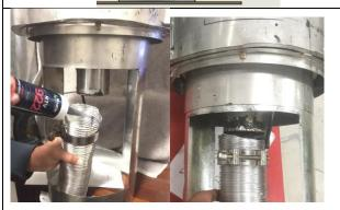
On the termination end - Fit clamp loosely & apply silicon inside the pipes. Apply an 8mm silicon bead fully around the inside of the flue and on the flue spigot. Smear smoothly around the surfaces.
