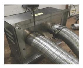
Feed air intake flue pipe through location spigot and fit retaining screw.
