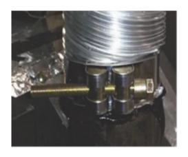
Slide flue onto connection spigot fully. Tighten clamp fully. Wipe excess silicon, visually check connection to ensure connection is fully sealed.
