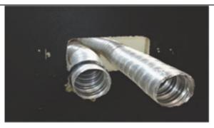
Cut flue exhaust tube (hot tube) to length (approximately flush with wall exit). Wall termination will sit against wall.
